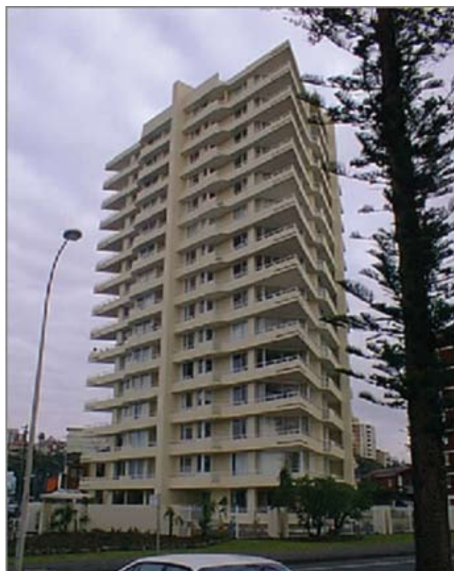
Figure 3: Cathodic Protection applied to the Trident building in Manly in 1997 (first application of CP to a residential building in Australia).
