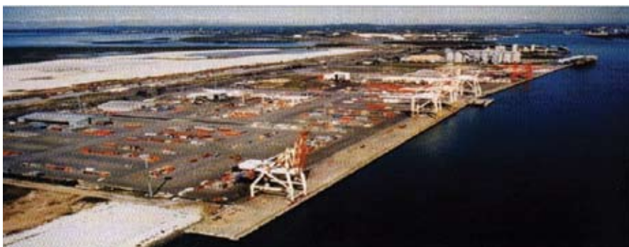
Figure 4: Cathodic Protection applied to Wharves 4 and 5 at the Port of Brisbane (completed in 1997)
