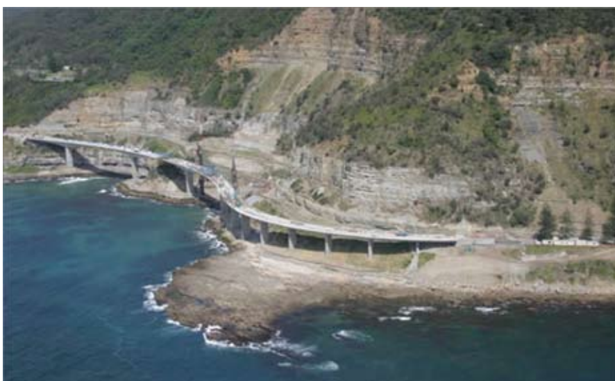
Figure 5: Cathodic Prevention applied to Seacliff Bridge, Lawrence Hargrave Drive, in 2005.
