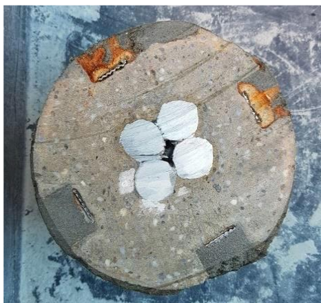
Figure 1. Grout acidification evident at anode locations
